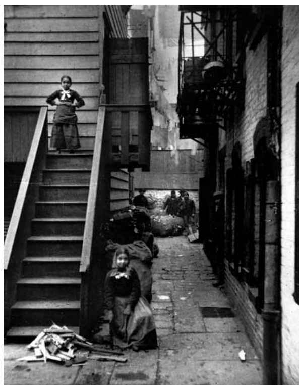
The entrance to a rear tenement building.
